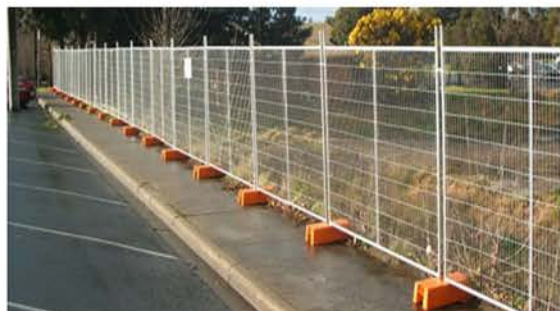
TEMPORARY FENCING WITH SHADECLOTH
